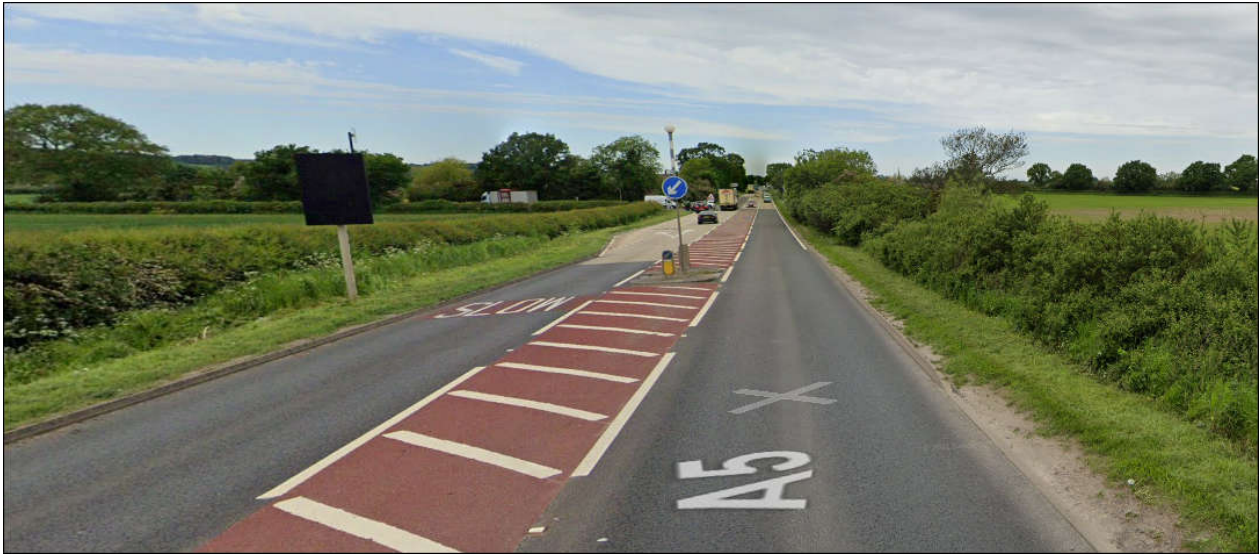
Figure 4-15: A5 Watling Street/Woodford Lane Junction Highway Safety Scheme
